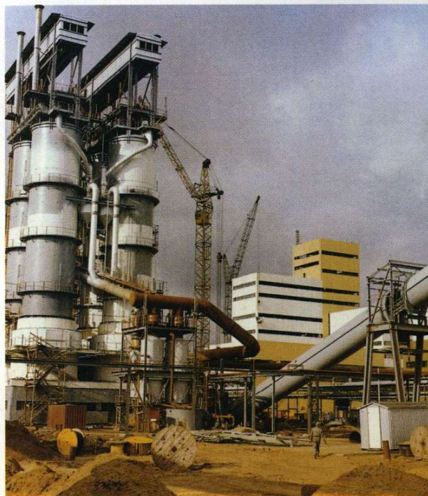
Dense Soda Ash Plant Inowroclaw/Poland Output: 3 x 550 t/24 h Particle size: 0,2 – 1 mm
